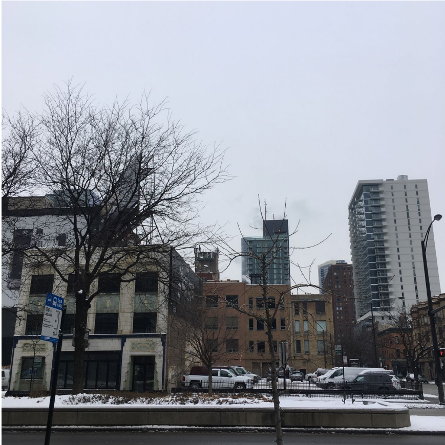
EXISTING PHOTO - LOOKING WEST
