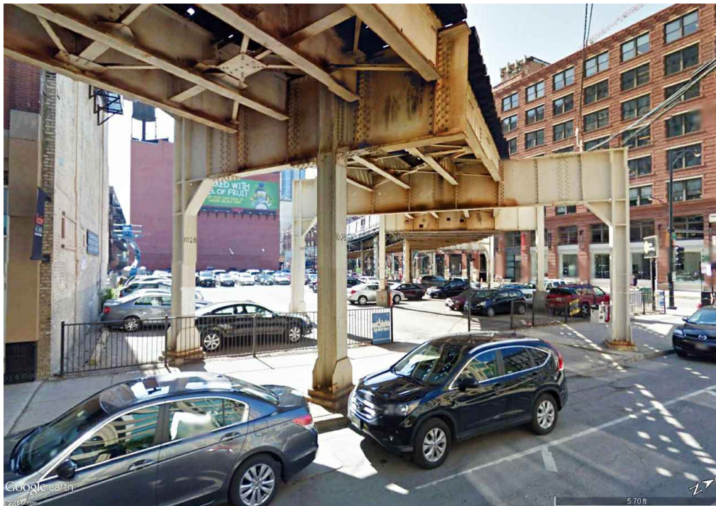
4) VIEW WEST ACROSS CTA SITE TOWARDS 225 WEST HUBBARD
